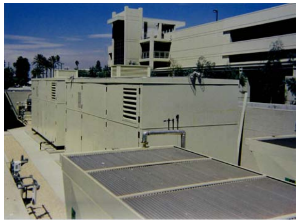
Kaiser Hospital Riverside, CA 2-200 kW Fuel Cells
